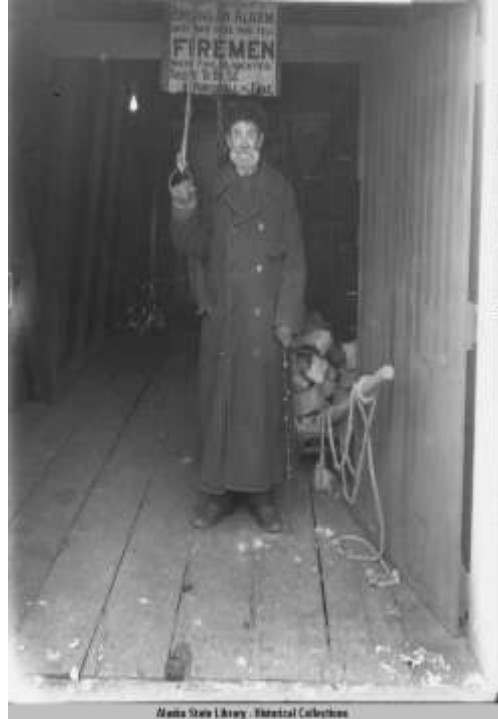
Daniel Kennedy holding the rope to the fire alarm bell—1900.
