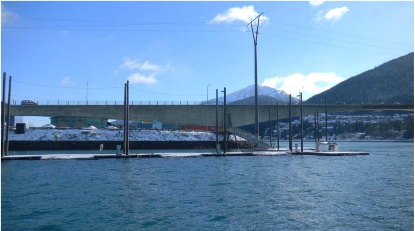
View of existing float at Bridge.
