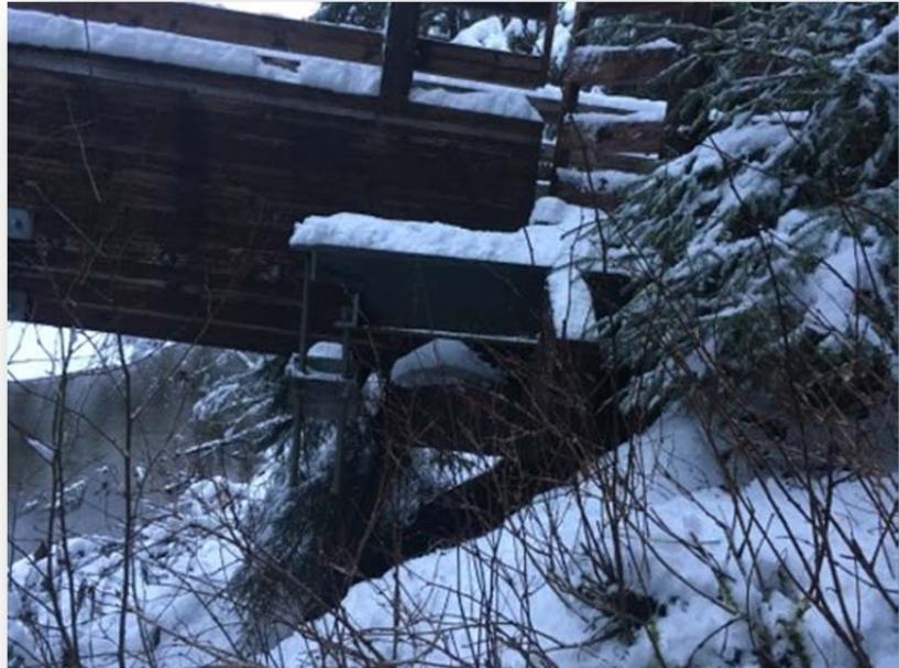
Recent photo of erosion under Montana Creek Bridge- the north end is now supported by metal beams as the foundation beneath the bridge has eroded away completely
