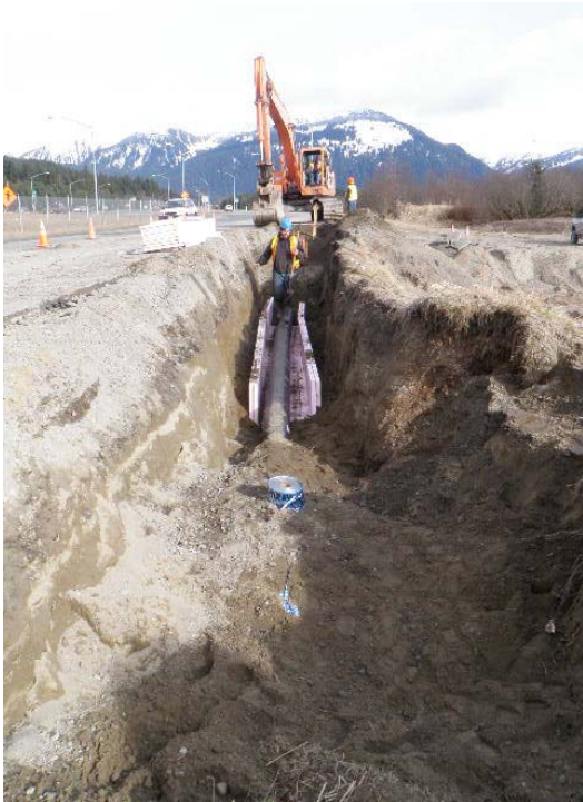
Water main installation at Maplesden Way
