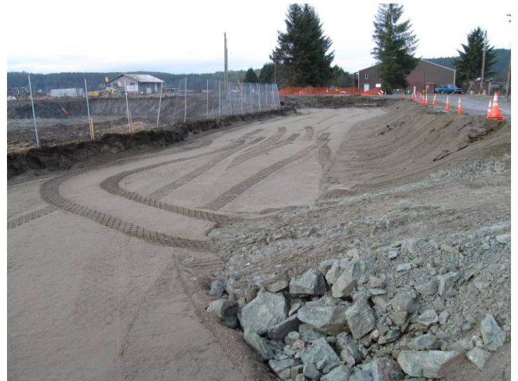
EVAR parking lot construction
