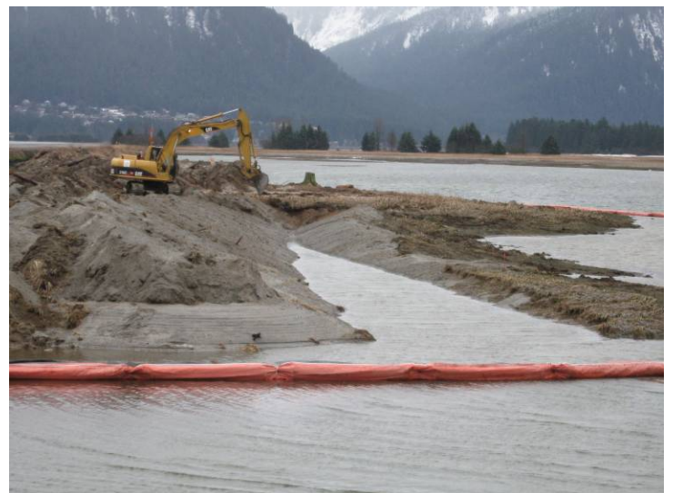
Lateral RSA silt curtain work
