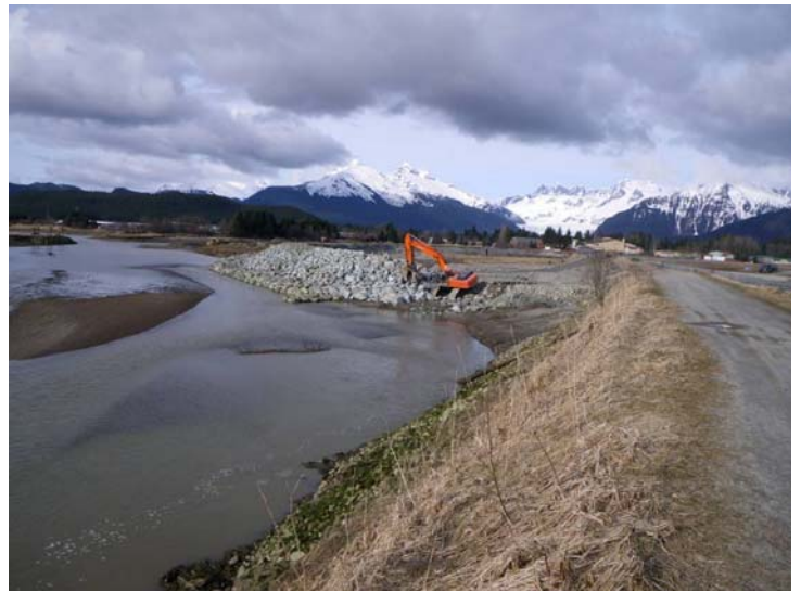
West end RSA rip-rap wall
