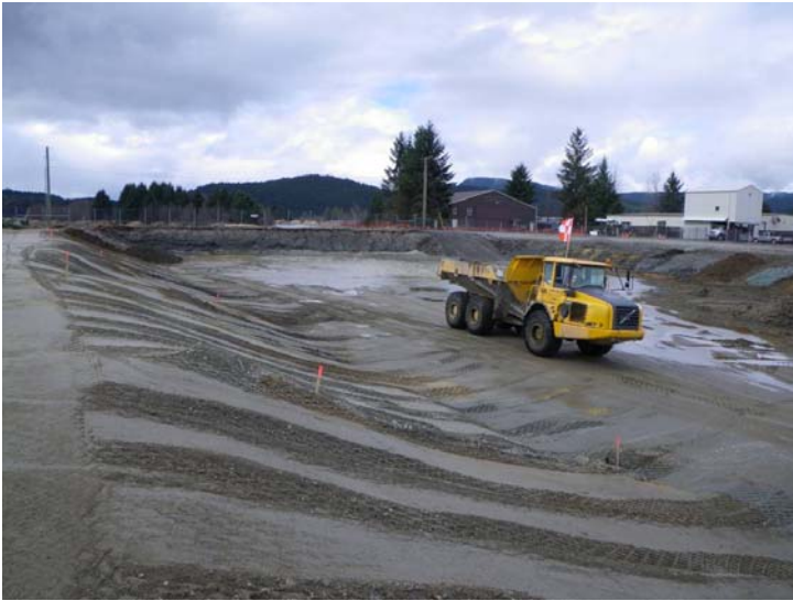
Duck Creek corridor excavation
