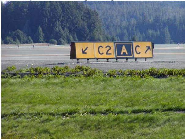
Taxiway Direction Sign sample
